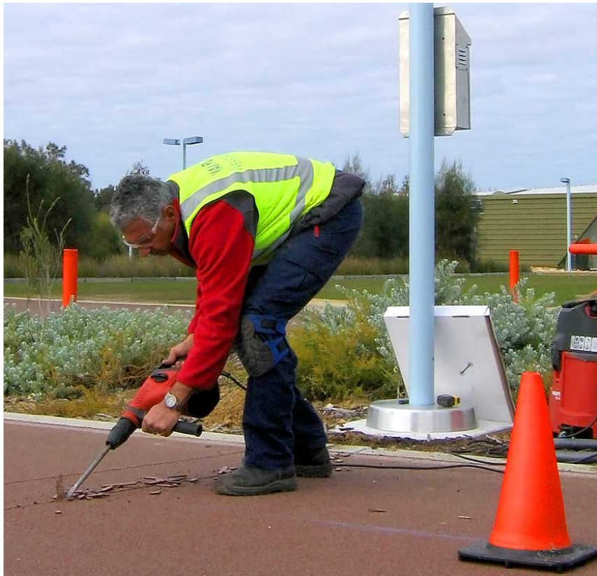
Chiselling out the slots
