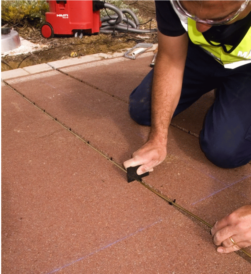
Inserting the piezo sensors
