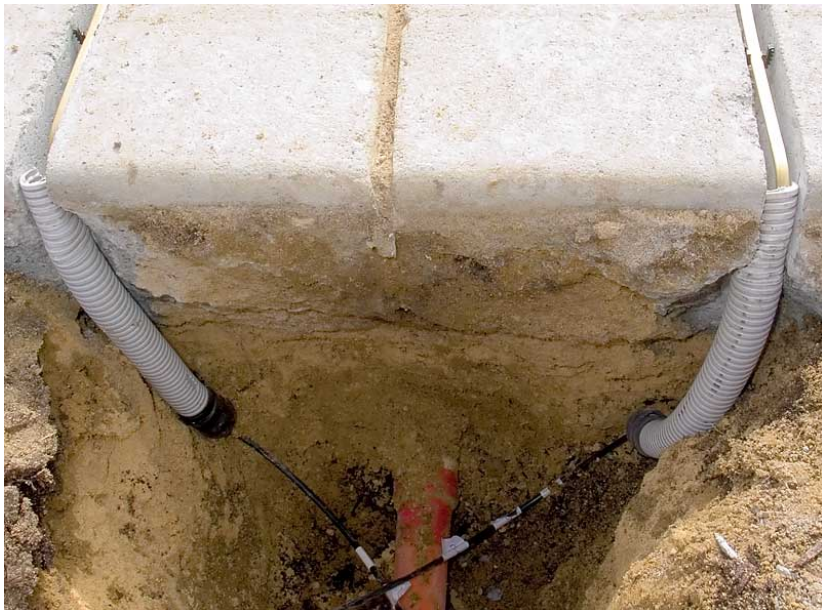
Cable routing detail
